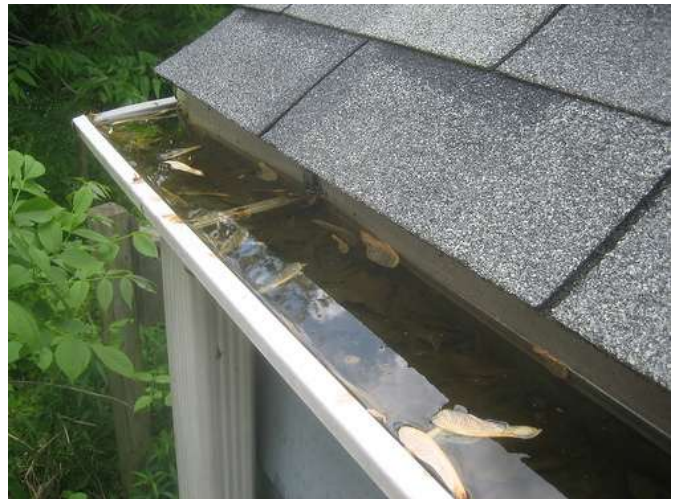
Figure 8. Clogged rain gutter filled with water
