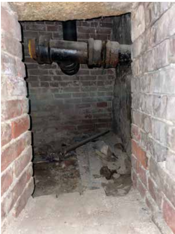
Figure 3.119 Cast-iron piping at original public restroom.
