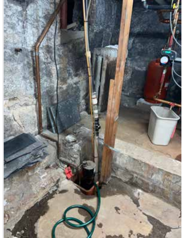
Figure 3.118 Basement boiler room - sump pump pit and pump.
