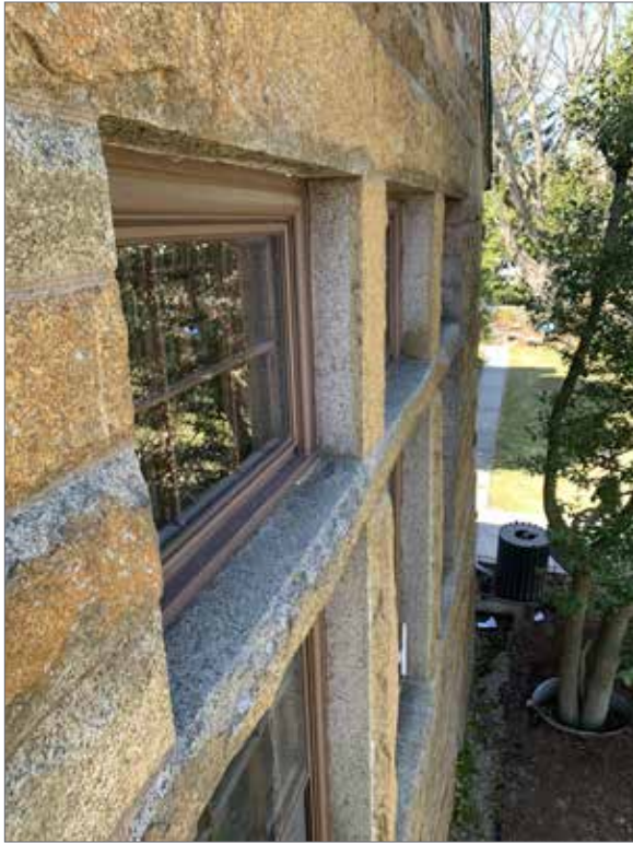
Figure 3.63 Detail - Rectangular fixed transom trim - 1exterior
