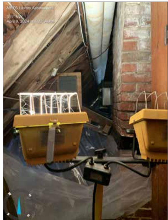
Figure 3.35G Rot damaged rafters in attic.
