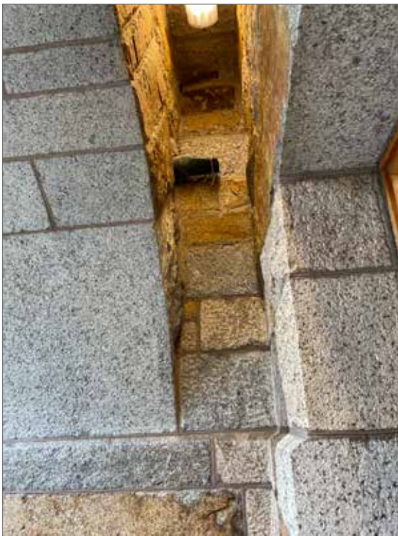
Figure 3.20 Lighting slot at arched main entrance.
