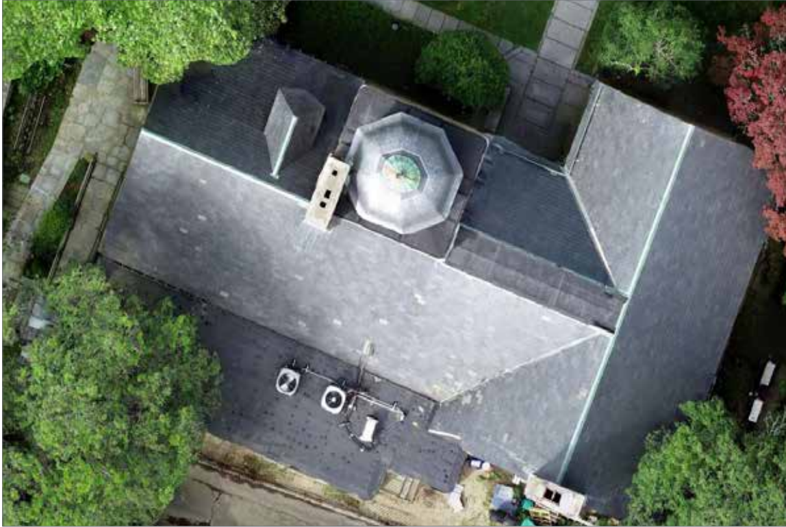
Figure 3.36 - Roof overview - aerial view - Note flat rectangular area to the right of side gable roof, between tower and intersection of end gable roof; this was the location of the skylight which was removed in the 1970s.
