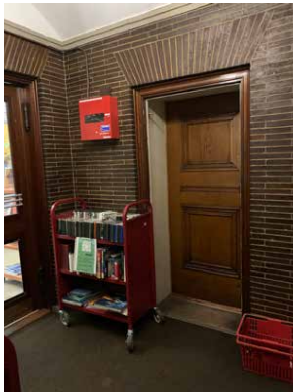
Figure 3.145 - Addressable fire alarm system panel. West wall of entrance lobby.. ..
