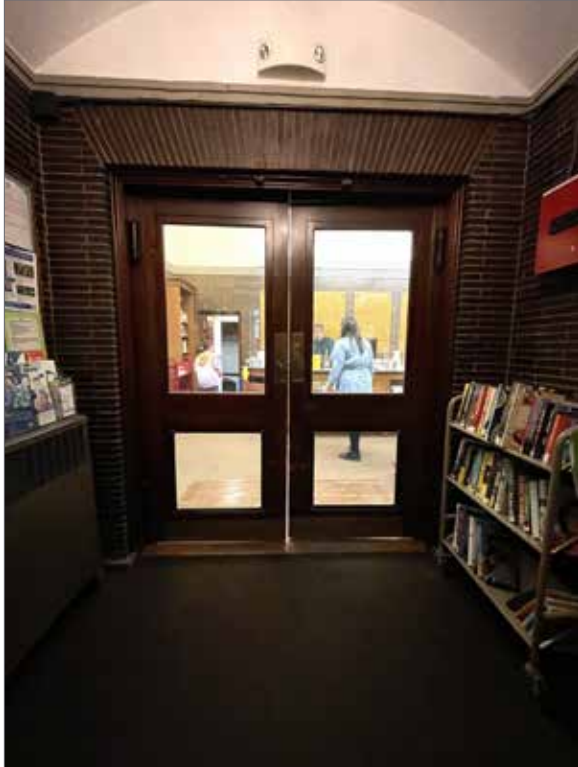
Figure 3.73 Main entrance hallway - interior two-lite double doors.
