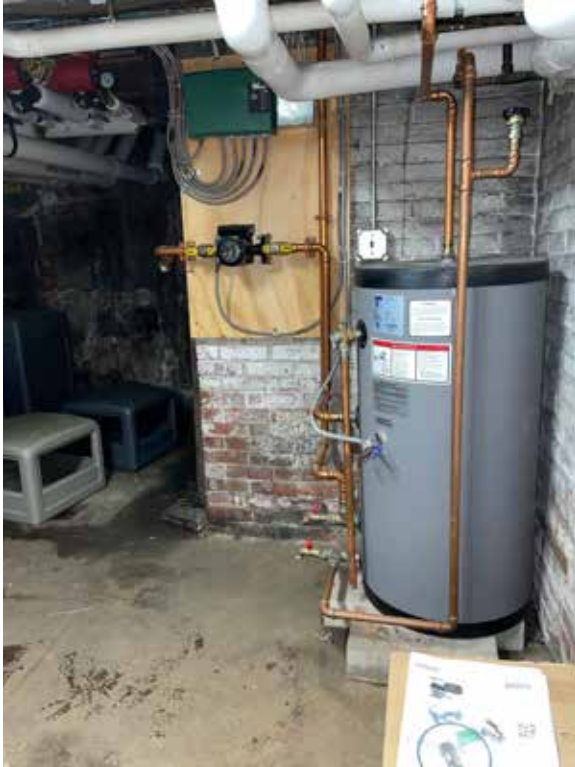
Figure 3.117 Basement boiler room - hot water heater.
