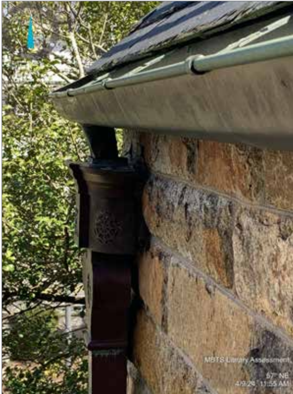
Figure 3.52 Original decorative rainwater conductor head, west elevation of end gable (library) roof.
