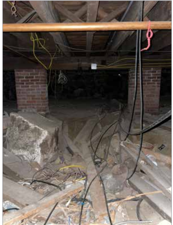
Figure 3.31 Brick piers and first floor wood framing under Library/Reading Room crawlspace - typical conditions
