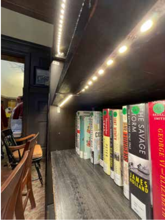
Figure 3.134 Under-cabinet lighting strip at underside of bookshelves in Library screen.
