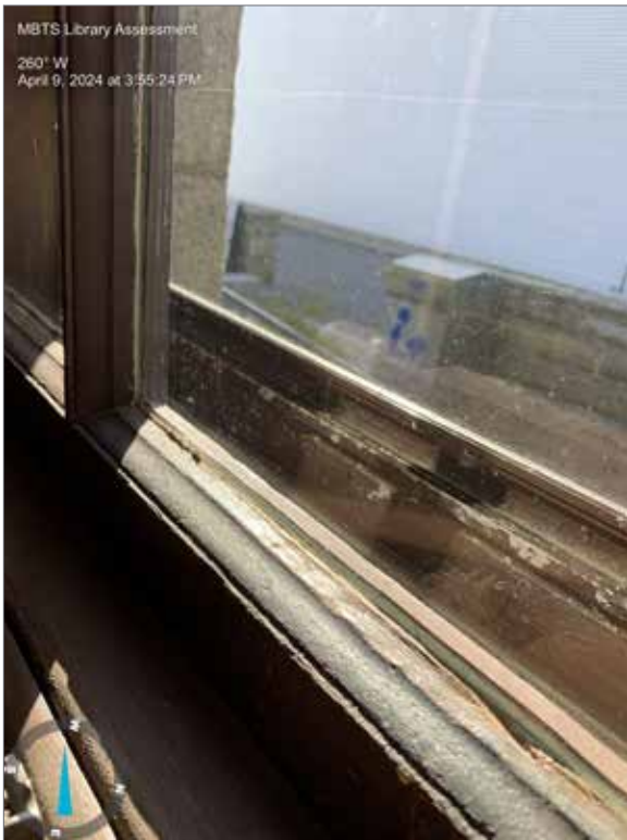
Figure 3.67 Single-hung windows == typical sash conditions.
