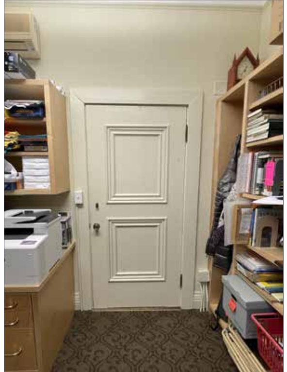
Figure 3.74 Interior paneled door - typical original paneling.
