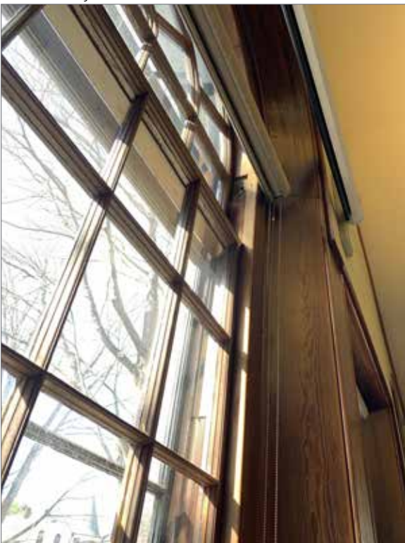
Figure 3.61 Detail at single-hung window with arched fixed transom above - interior.
