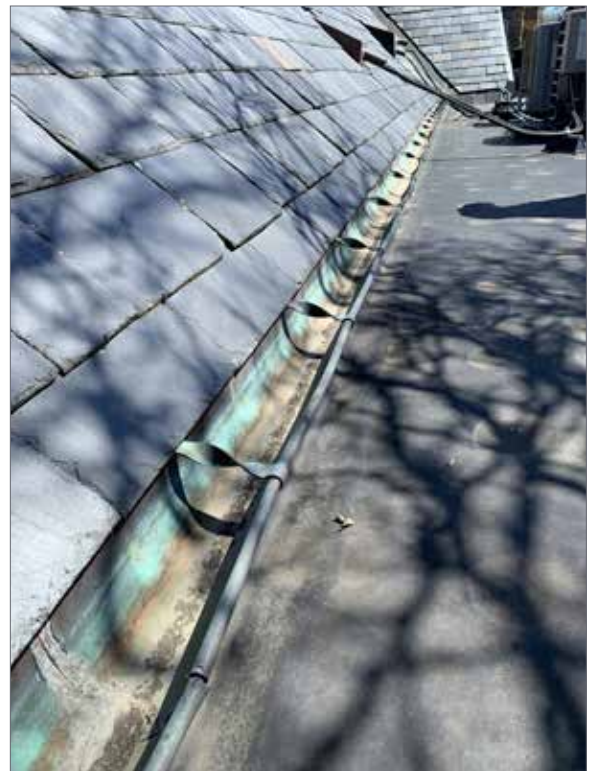
Figure 3.47 Replacement gutter at side gable roof - south elevation.
