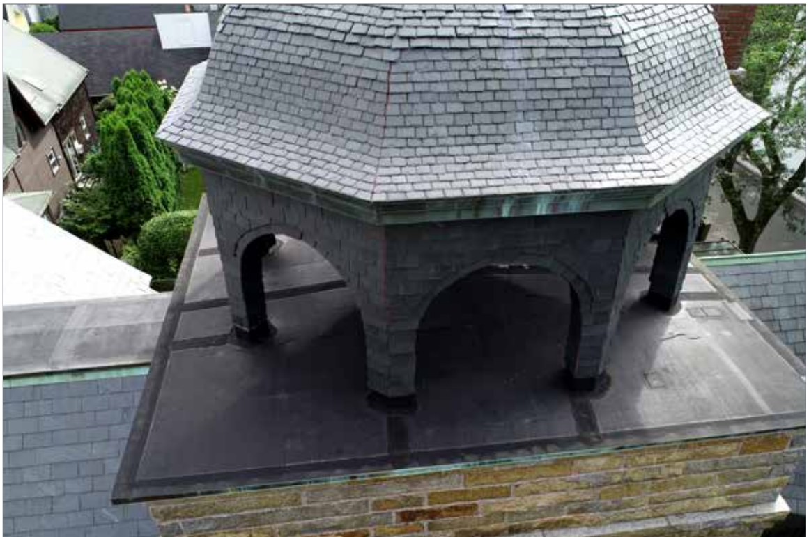
Figure 3.39 - Tower flat roof and slate clad cupola roof - aerial view from north looking south.
