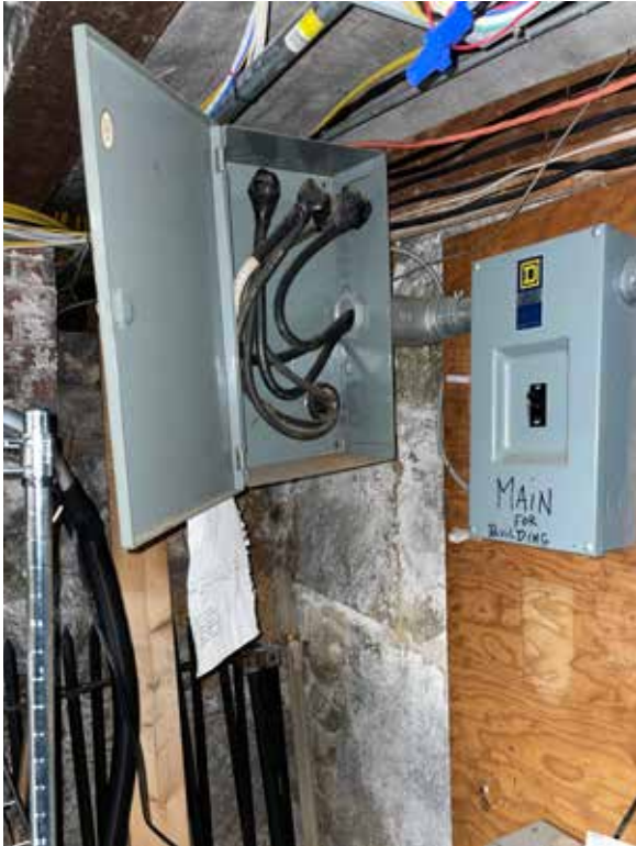
Figure 3.122 Main building enclosed circuit breaker.
