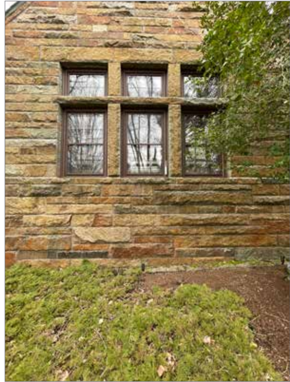
Figure 3.60 Triple single-hung operable windows with fixed rectangular transoms - typical exterior window finishes.
