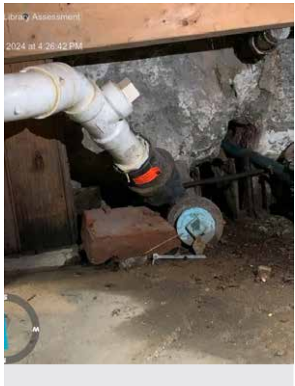
Figure 3.120 Cast-iron and new PVC piping at basement utility sink.
