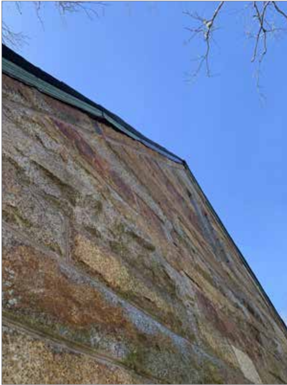
Figure 3.18 Field masonry at gable end."
