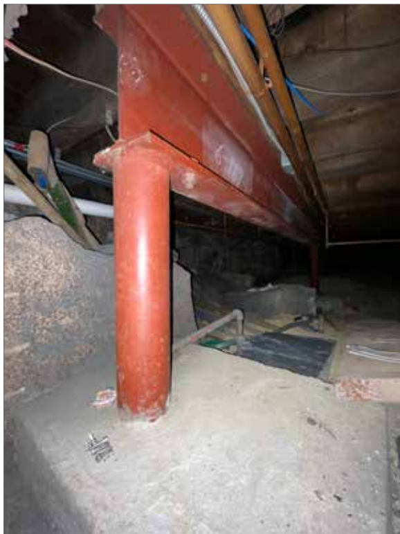
Figure 3.32 Steel structural reinforcement in GAR Hall/Reference Room crawlspace.
