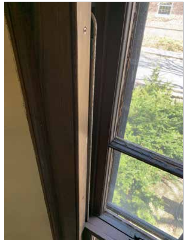
Figure 3.66 Typical single-hung window cable and pulley operating hardware.
