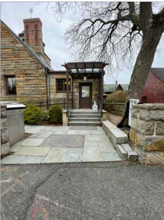
Figure 3.09 Bluestone paving and displaced retaining wall at west entrance
