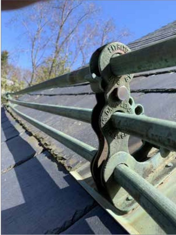
Figure 3.44 Original pipe snow-guard - detail.
