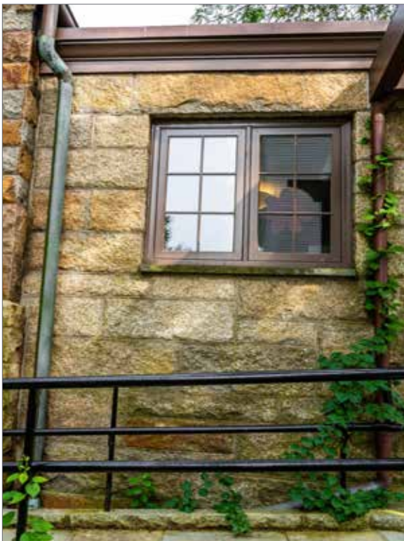
Figure 3.57 Children's Room Addition flat roof downspout - west elevation.
