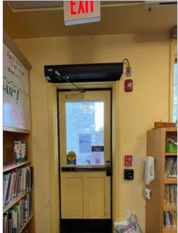
Figure 3.80 West entrance to Children's Room Addition - interior. Panic bar and barrier free access hardware..
