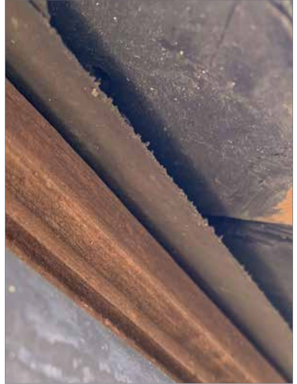
Figure 3.45 Edge of cut original high-back gutter under starter slate - east elevation of library roof.
