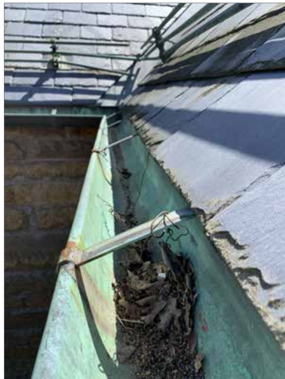
Figure 3.43 Original copper high-back gutter and pipe snow-guard at main entrance.
