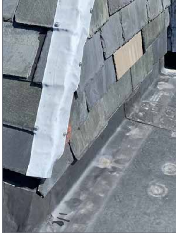
Figure 3.49 Flashing repair at south end of gable wall.
