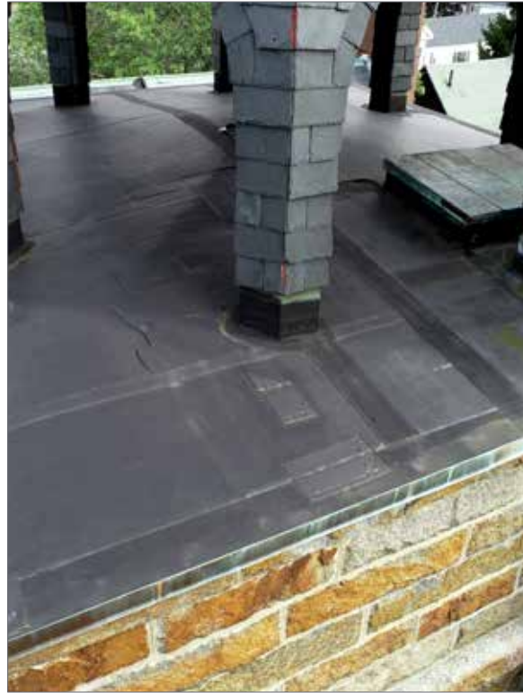
Figure 3.41 Membrane roofing at tower flat roof, sheet copper clad cap at access panel beyond.
