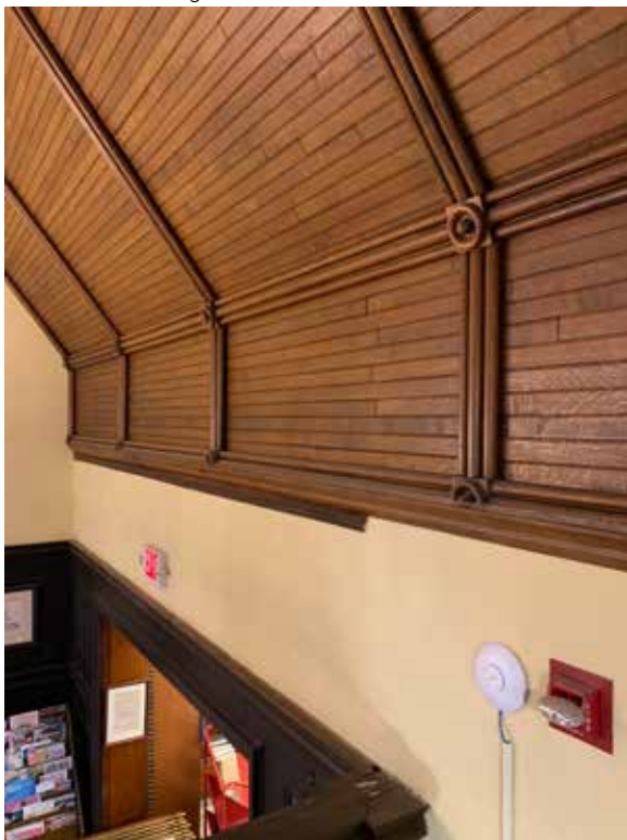
Figure 3.101 Original oak paneled vaulted ceiling. Library/Reading Room, view from upper stacks Teen Loft.
