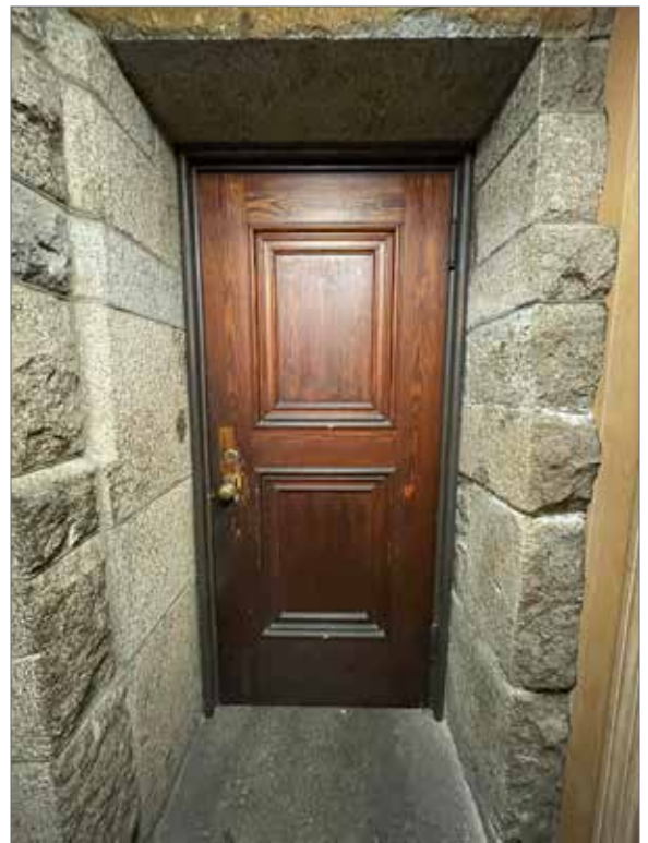
Figure 3.21 Masonry opening - Staff Restroom.
