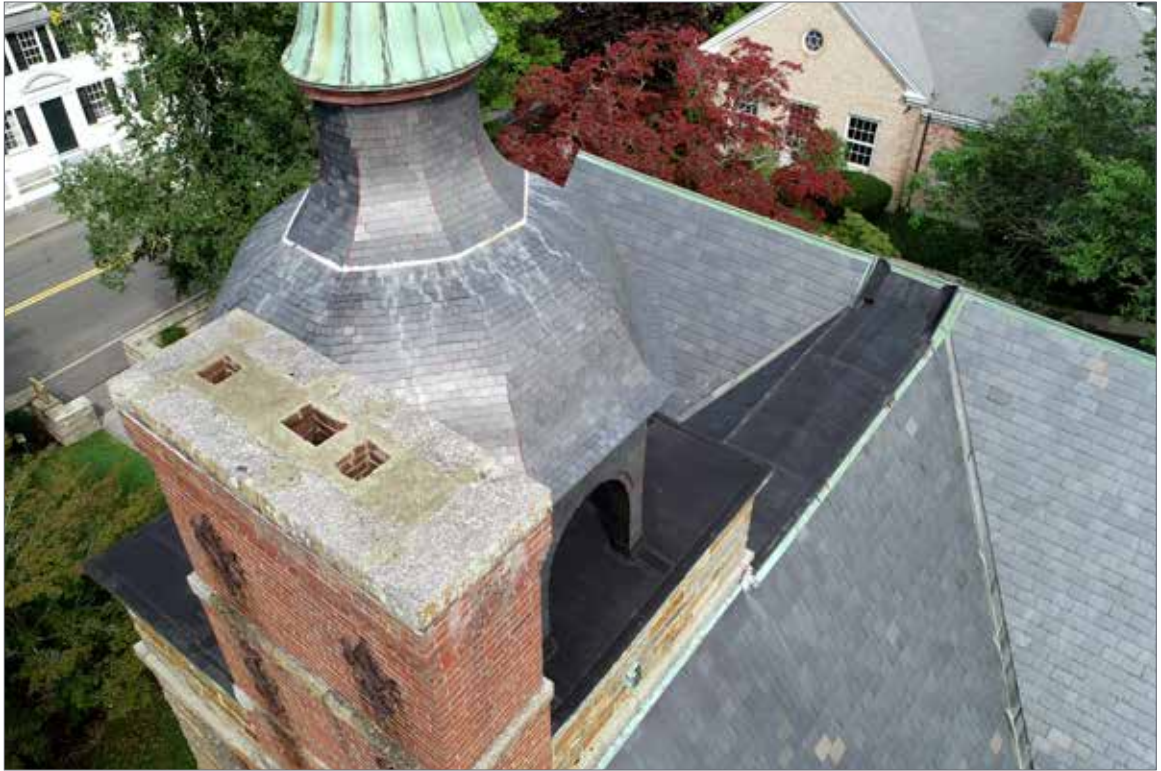
Figure 3.38 - West chimney (forefront), cupola, intersection of end gable and side gable roof, and membrane roofing at flat area where skylight used to be located. Aerial view from west looking east.."
