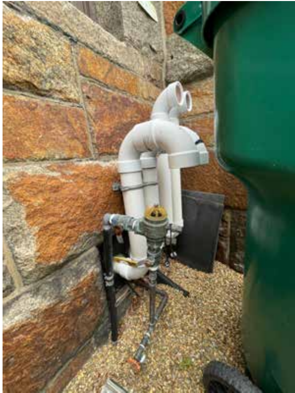
Figure 3.110 Boiler exhausts
