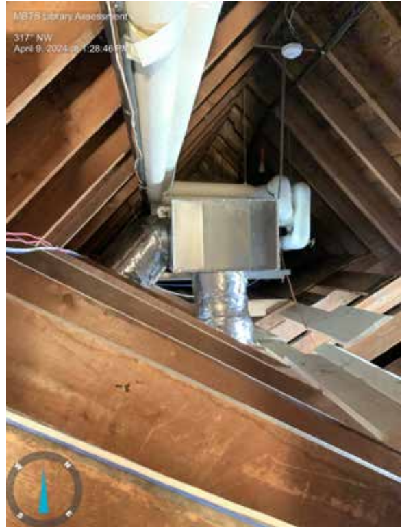
Figure 3.111 - Ductwork and vent - attic above side gable wing, near dormer.
