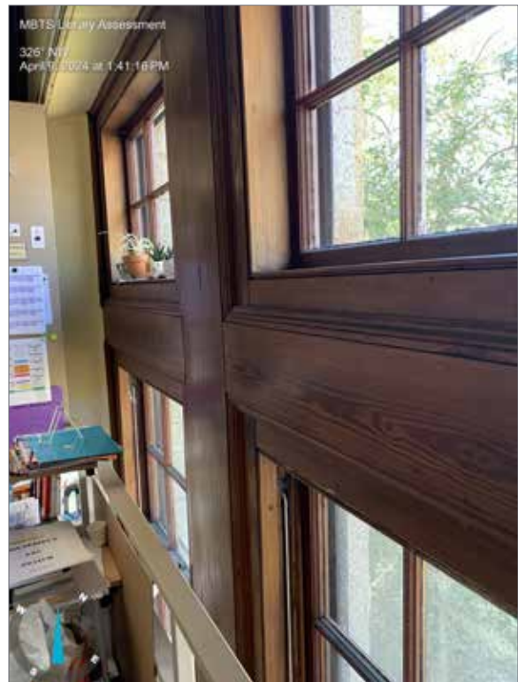
Figure 3.62 Detail at single-hung window with fixed rectangular transom above - interior.
