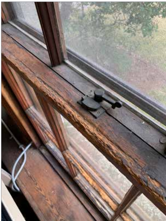
Figure 3.65 Typical single-hung window closing hardware and sash conditions..
