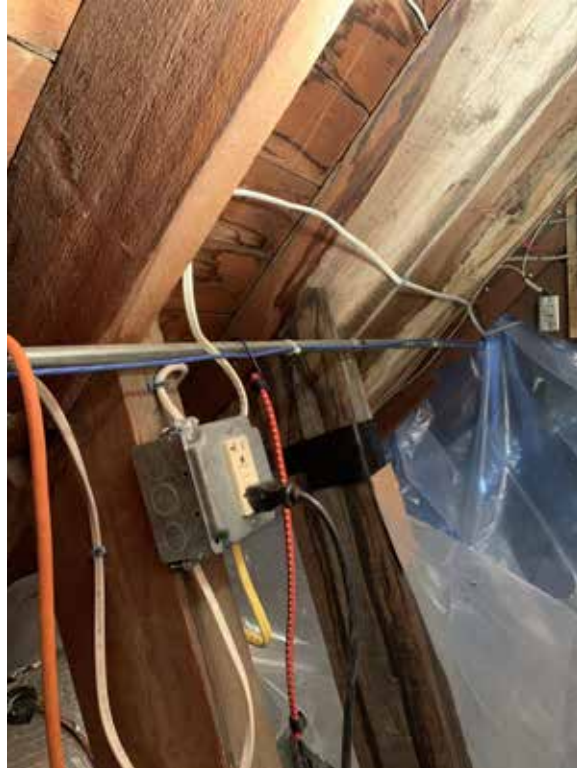
Figure 3.127 - Wiring and outlets in attic..
