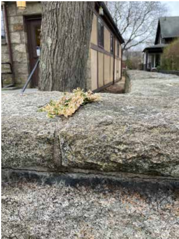
Figure 3.05 Perimeter wall - vegetation growth
