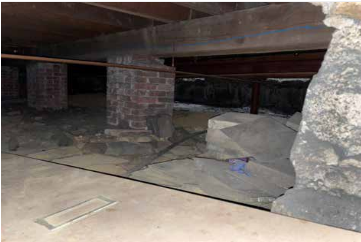
Figure 3.35B - Brick piers and first floor wood framing under GAR Hall/Reference Room crawlspace - typical conditions
