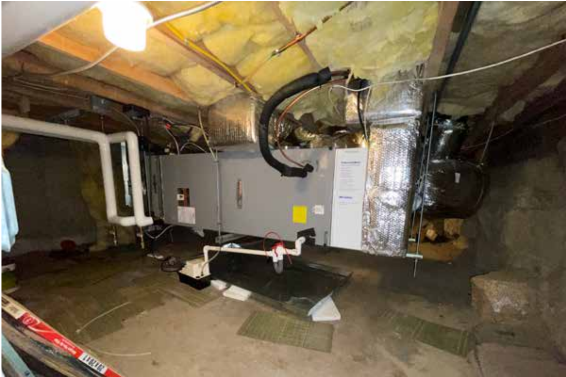
FIGURE 3.114 - Children's Room Addition - unit in crawlspace.
