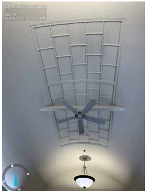
Figure 3.102 Original framing of closed skylight at Memorial Hall/Circulation Room.
