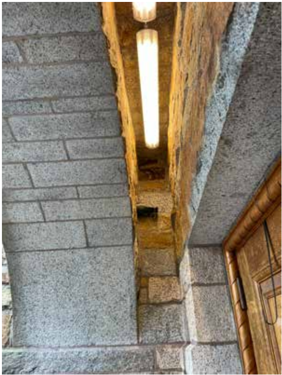
Figure 3.148 Exterior - Indirect lighting at main entrance.
