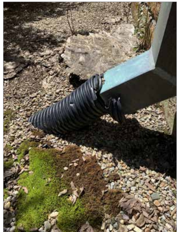
Figure 3.55 Downspout to grade.
