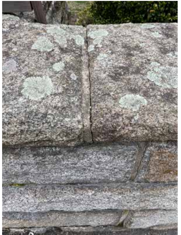
Figure 3.06 Perimeter wall - biological growth.
