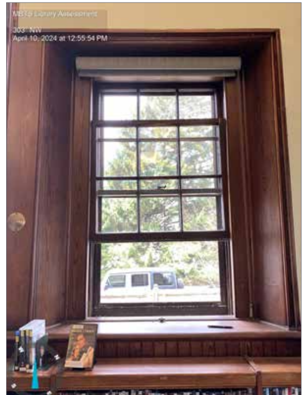
Figure 3.64-Typical single-hung window - interior
