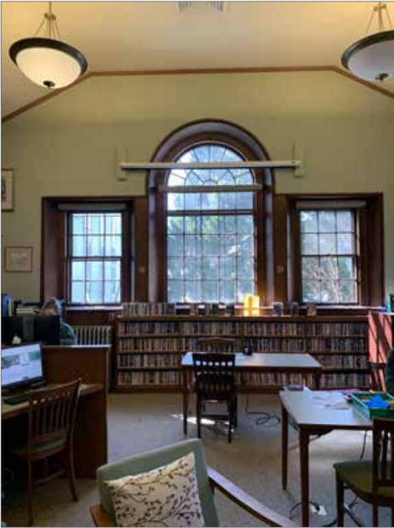
Figure 3.59 Triple single hung operable window, with central arched fixed transom - typical interior finishes
