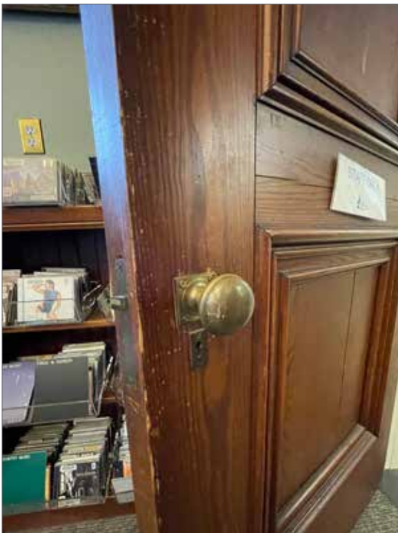
Figure 3.77 Original interior door - typical paneling and hardware.
