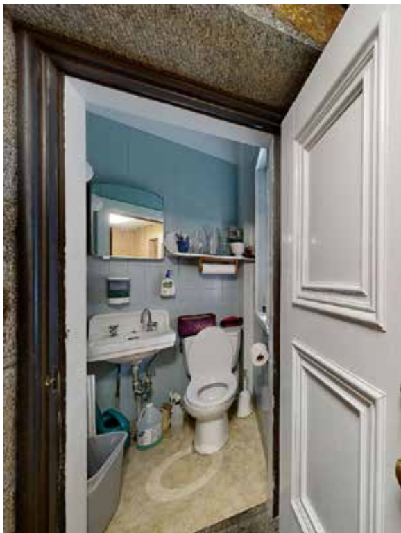
Figure 3.97 Plaster ceiling, ceramic tile wall finish, vinyl sheet flooring, wood trim. Staff restroom.,
