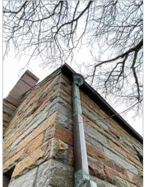
Figure 3.53 Rainwater conductor head and downspout, southeast corner of end gable (library) roof.
