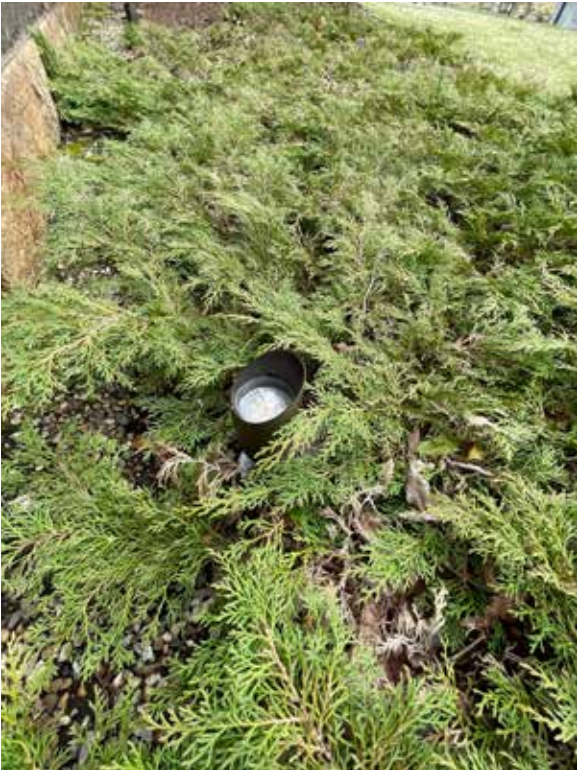
Figure 3.147 -Exterior uplighting fixture
