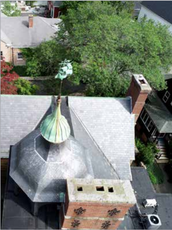
Figure 3.40 Chimney caps and weather vane.
