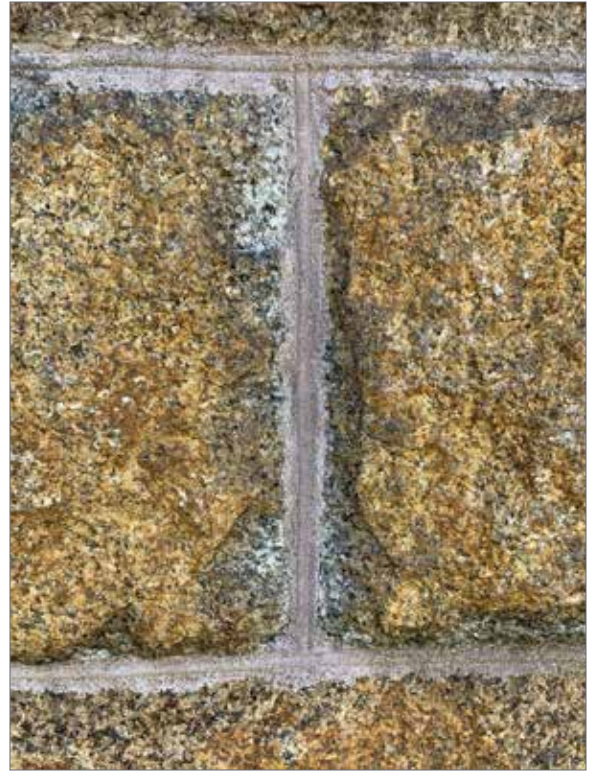
Figure 3.19 - Granite masonry mortar joints."
