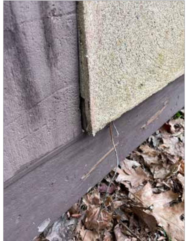
Figure 3.27 South elevation - stucco panel displacement.
