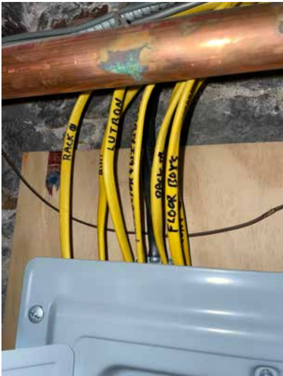
Figure 3.125 Labeled cables from distribution panel.
