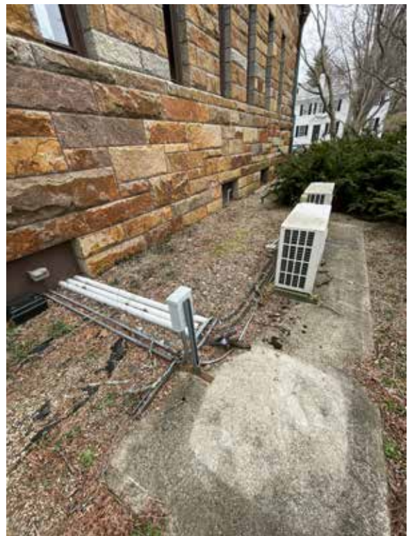
Figure 3.113 Decommissioned exterior units.
