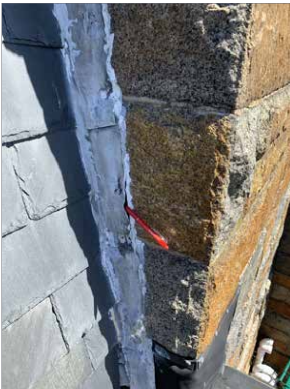
Figure 3.46 Damaged wall copper flashing repair. Note multiple layers of sealant repairs.
