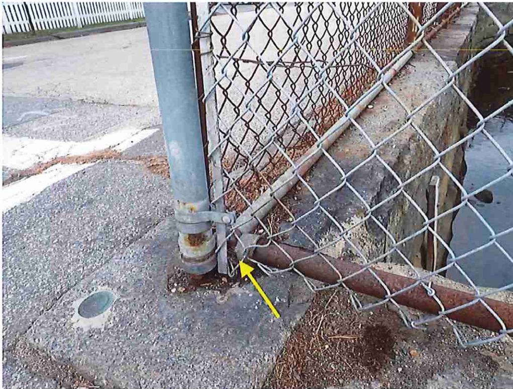
Photo 5: Bottom rail detached from the west post on the north fence.
