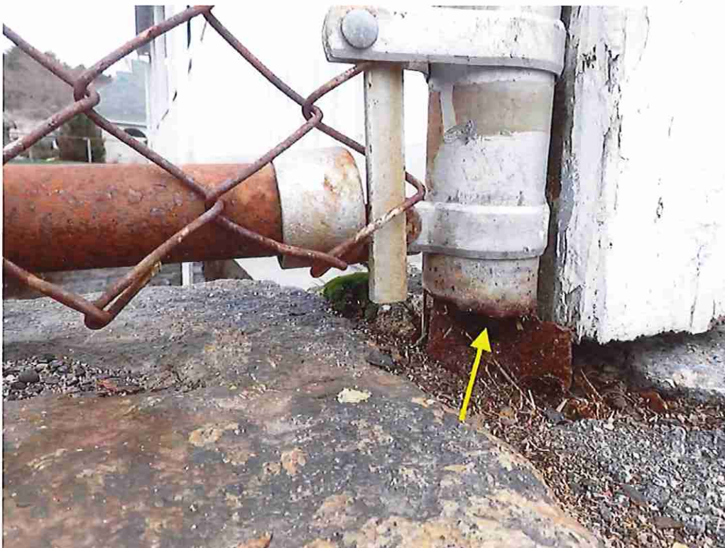
Photo 4: 100% section loss to the east post on the north fence.
