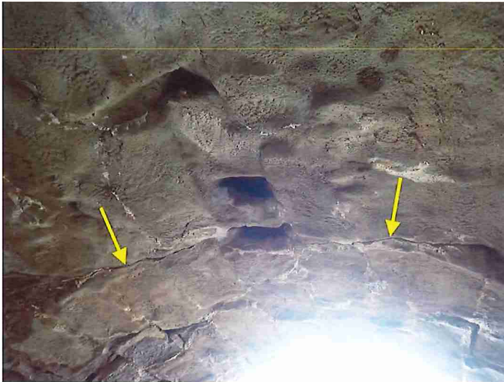
Photo 7: Full length crack in the arch at 7' from the south fascia and voids in the keystone area.
