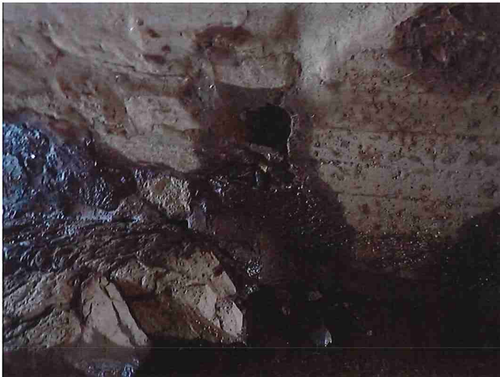
Photo 6: Void in the arch at 18' in from the north fascia, 3-1/2' above the west spring line.
