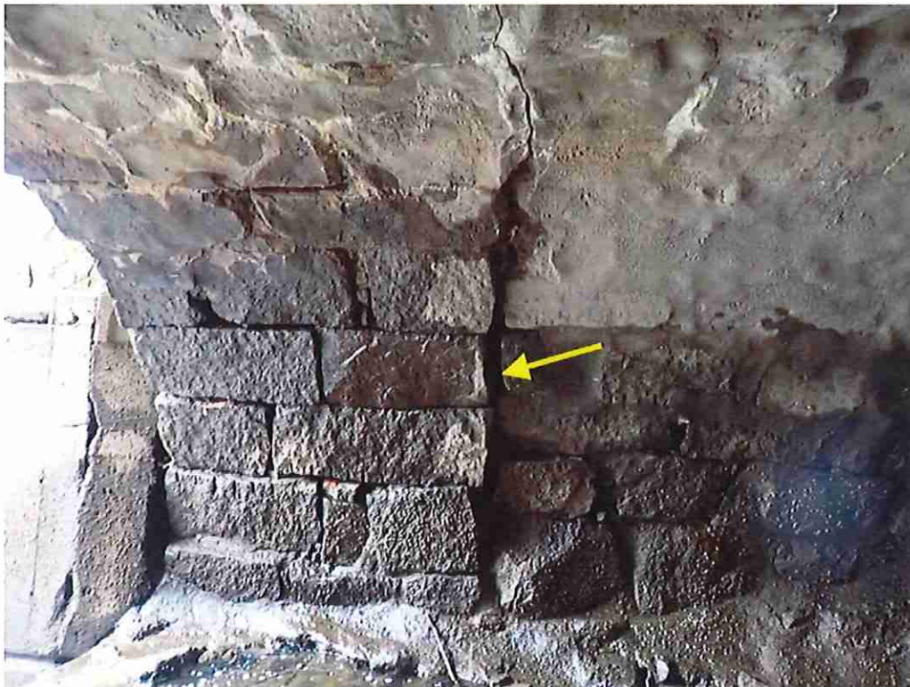
Photo 8: Void above the west spring line at 7' in from the south fascia.
