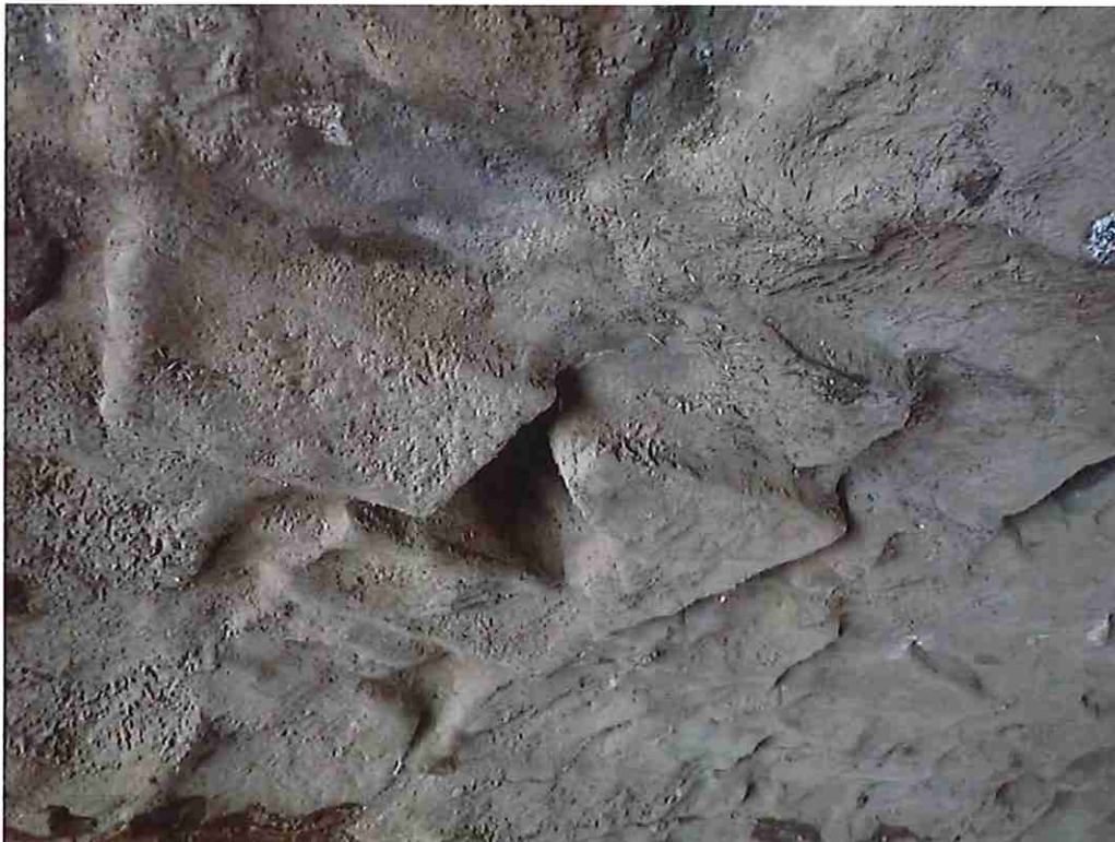
Photo 10: Void in the keystone area at 14' in from the north fascia.
