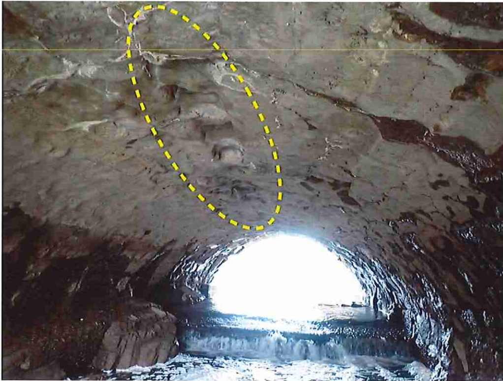
Photo 9: Typical voids and unevenness throughout the keystone area.
