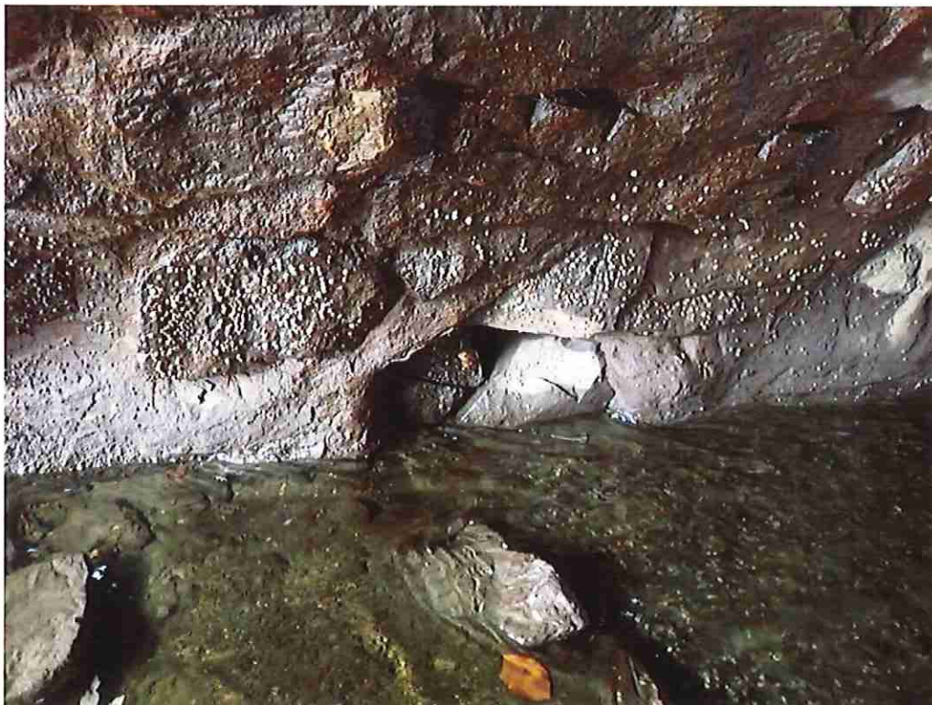
Photo 14: Void in the east spring line at 9' in from the north fascia.
