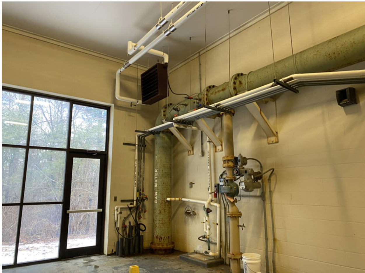
Figure 8: Entry of raw water piping into filtration room
