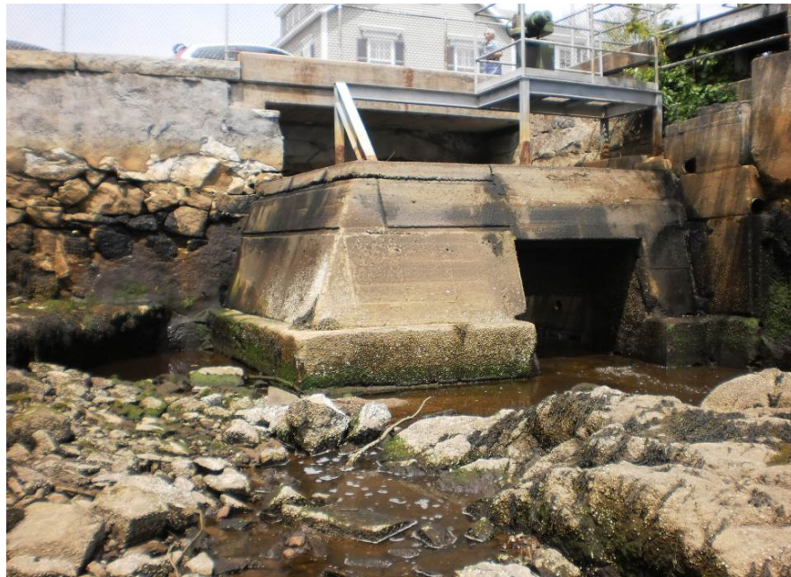
Figure 2.11 Tide Gate, Seawall, and Culvert Structures at Central Street
