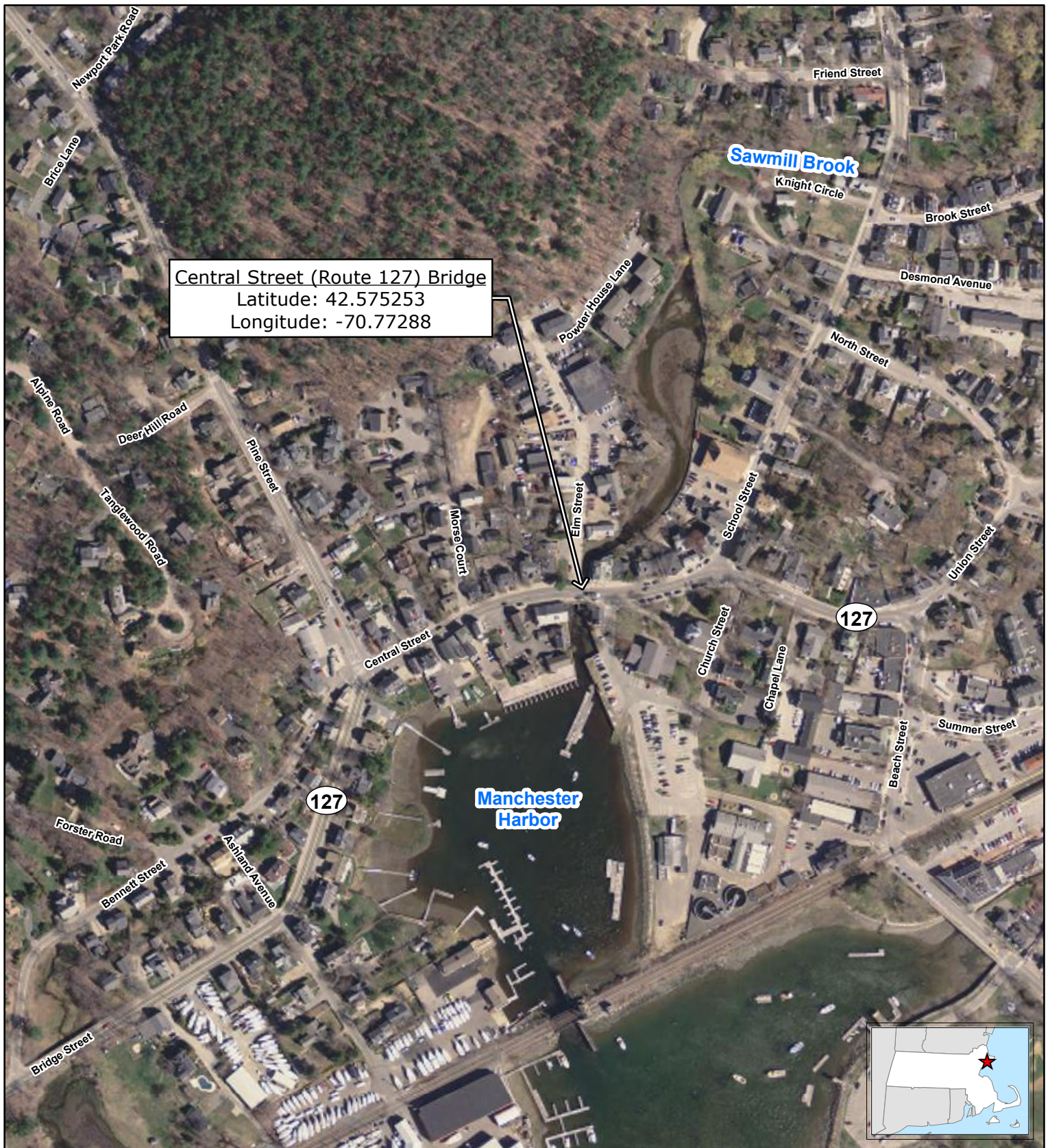
FIGURE 1 SITE AERIAL OVERVIEW
