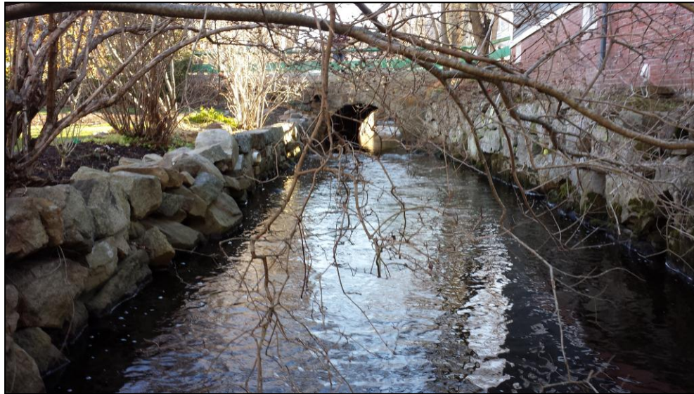
Outlet of School Street Culvert
