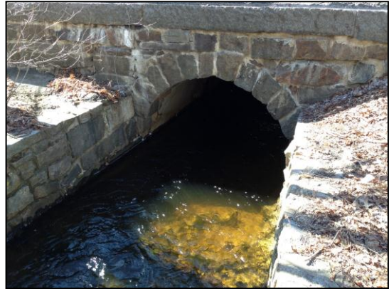
Inlet of School Street Culvert
