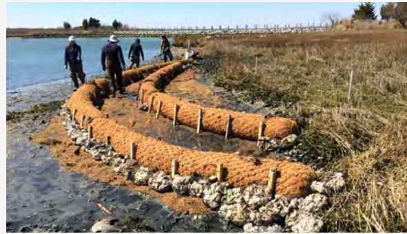
Oyster reefs stabilize the coast by acting as natural breakwaters that grow and change with the sea. In Rehoboth, Delaware, oyster restoration projects also provide a strong local economy. Source: DNREC Wetlands Monitoring & Assessment Program
