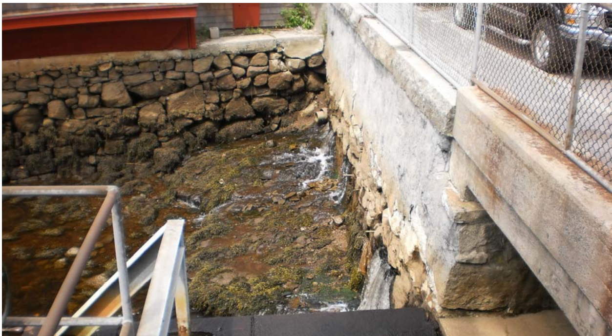
Photo 1 Water seepage (flow) coming from the stone culvert side wall
