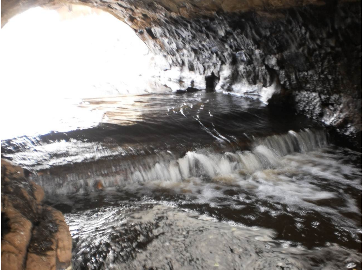
Photo 7 Mid length weir inside culvert, bedrock left
