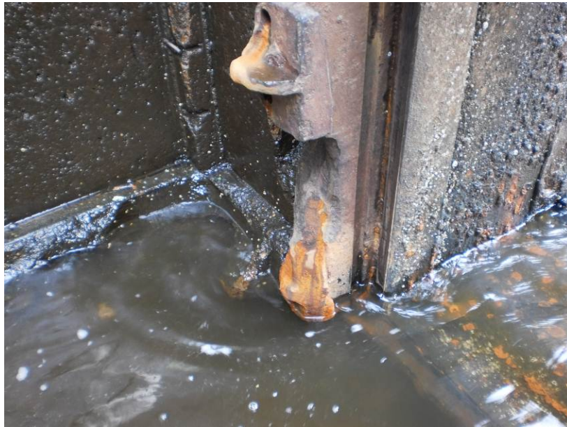
Photo 2 Corrosion/erosion of low tide gate tracks
