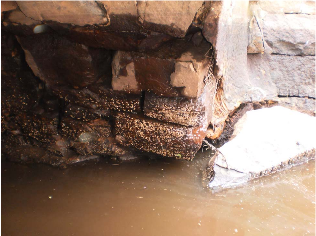
Photo 3 Northwestern corner arch stones unsupported
