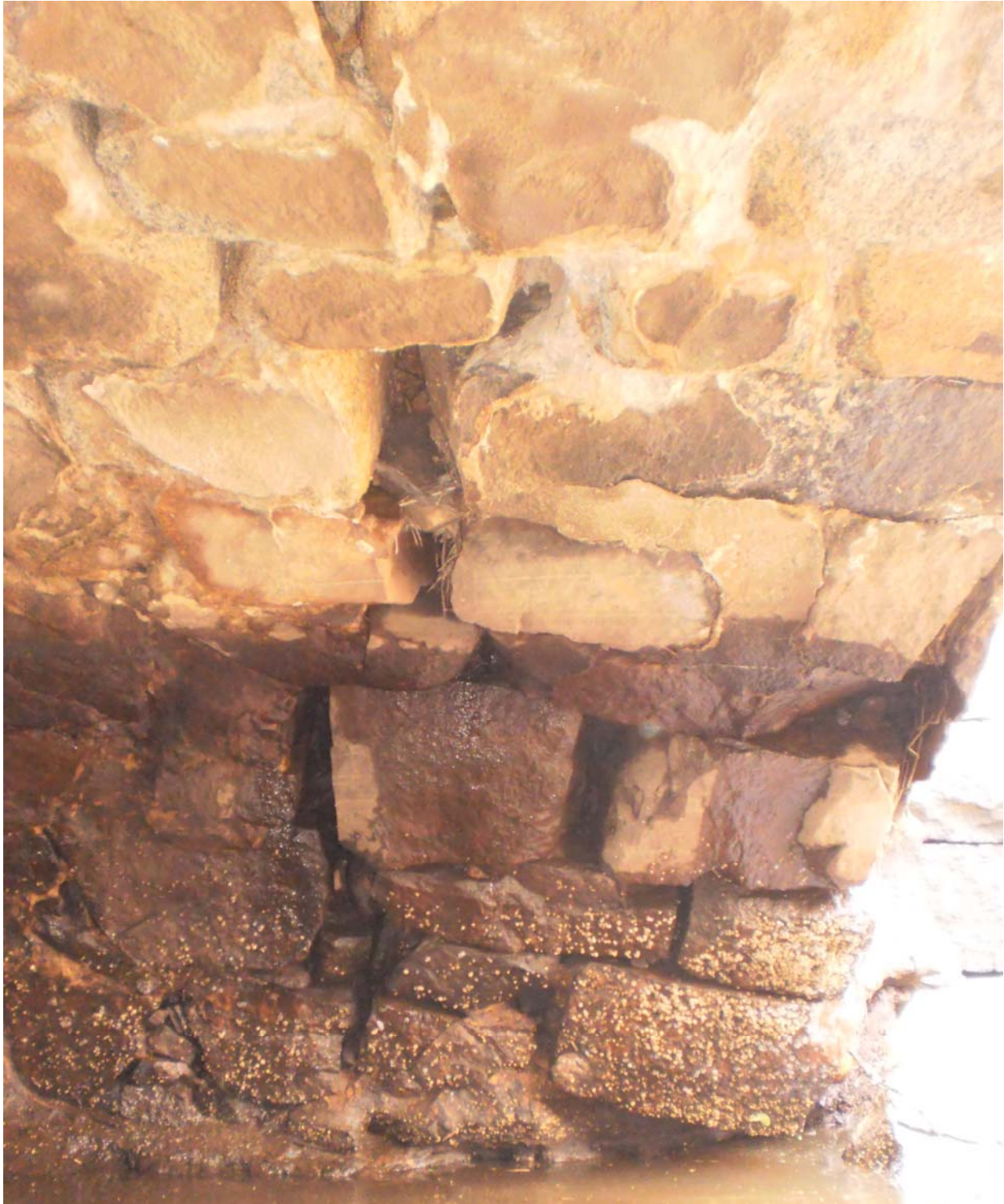
Photo 2 Separation and settlement of culvert arch stones, upstream, northwestern corner
