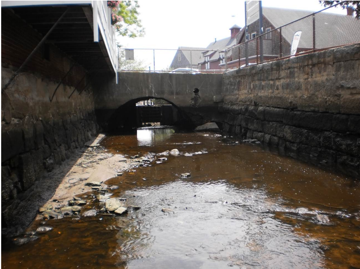
Photo 9 Stream channel upstream from culvert looking south with dark staining on walls indicating normal gate closed high water level
