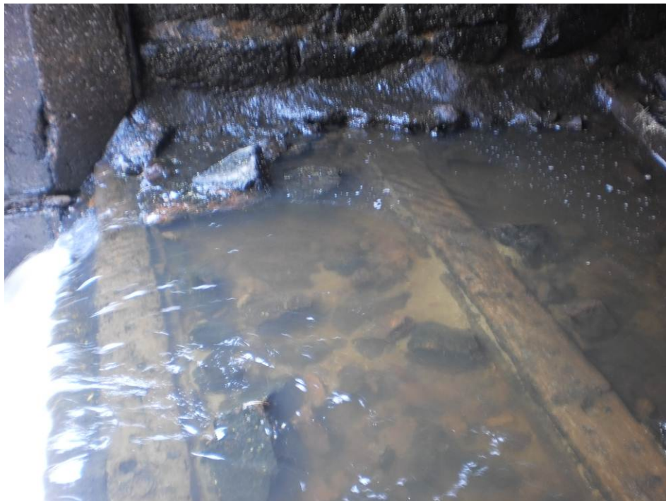
Photo 6 Apparent rock filled timber cribs forming stream bed at south end of arch culvert
