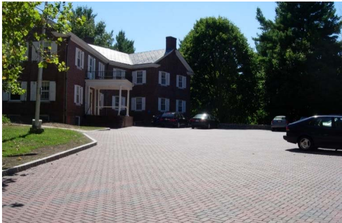
Figure 6 Permeable paver parking, University of New Hampshire, Durham, New Hampshire
