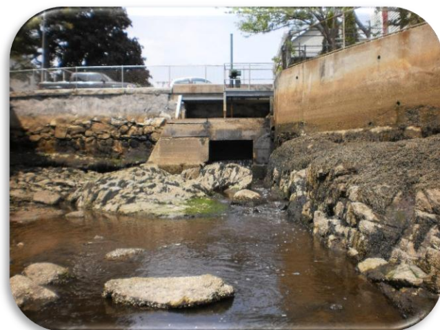
Bedrock configuration downstream of tide gate
