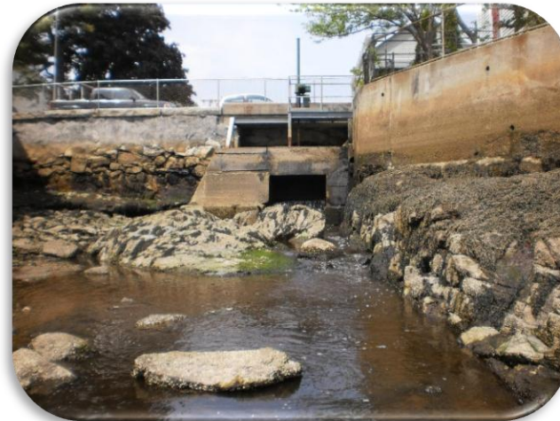
Bedrock configuration downstream of tide gate
