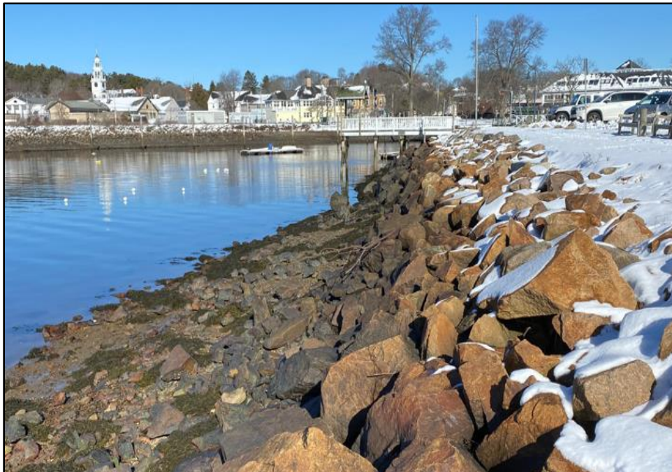
Figure 13. Cobbles and boulders along the toe of sloping rock revetment along northern slope of Masconomo Park. Feature is continuous with the toe of the coastal engineering structure and therefore not delineated as rocky intertidal shore. Photo taken facing east.
