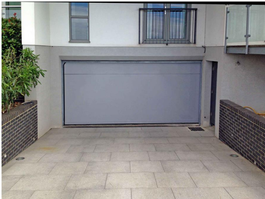
Floodproofed garage door (Image credit: Flood Control International)
