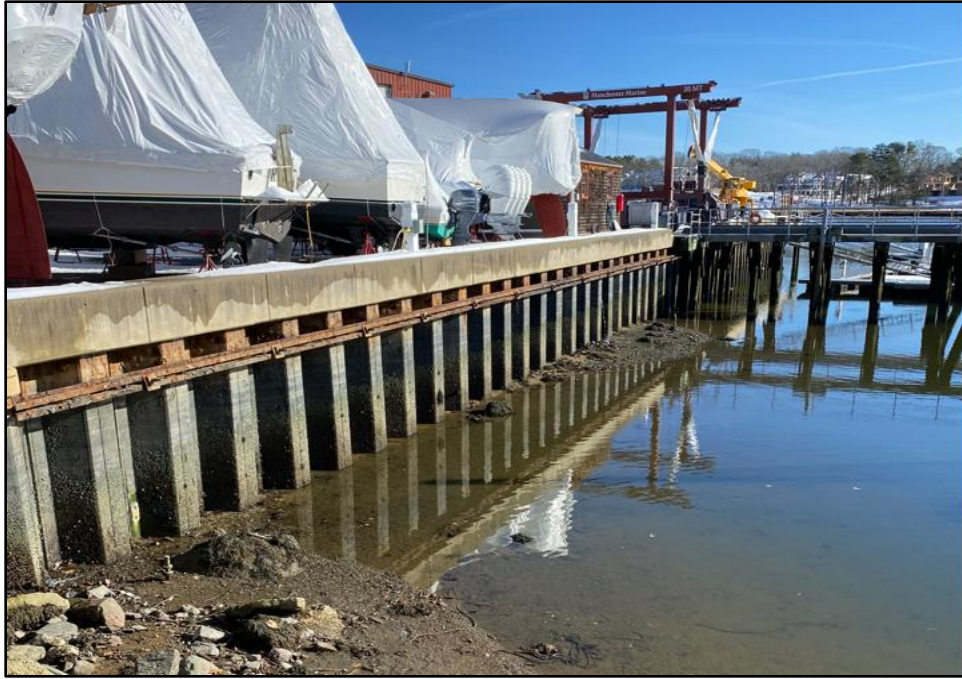
Figure 6. Vertical sheet pile bulkhead abutting Crocker's Boatyard. Photo taken facing northeast.
