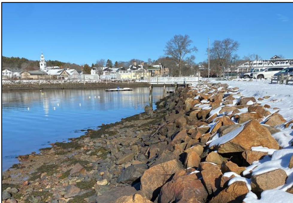
Figure 3. Sloping rock revetment along the northern shoreline of Masconomo Park. Photo taken facing northeast.
