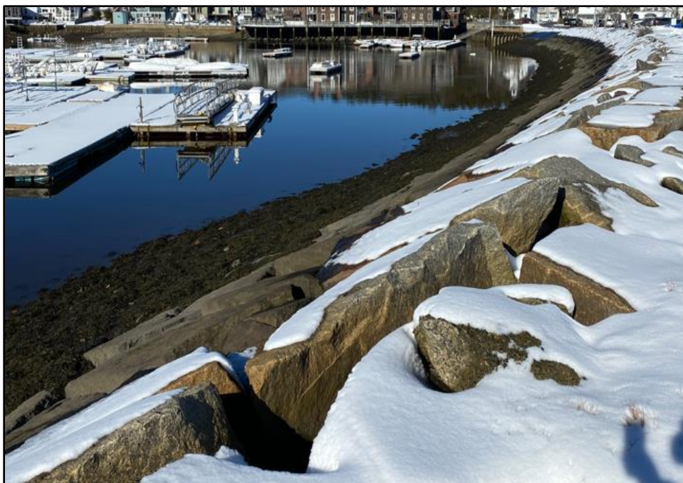
Figure 14. Visible macroalgae attached to boulder toe stones of sloping rock revetment in upper basing of Manchester Harbor. Note – this area was not delineated as rocky intertidal shore. Photo taken facing north.
