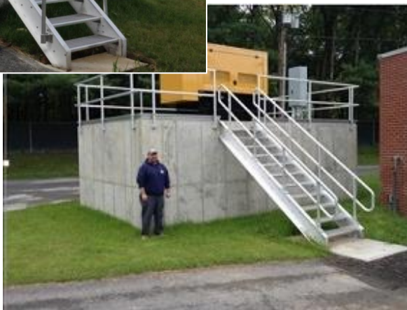
Elevation of standby generators (Image credits: FEMA and Magna Engineers, 2013)
