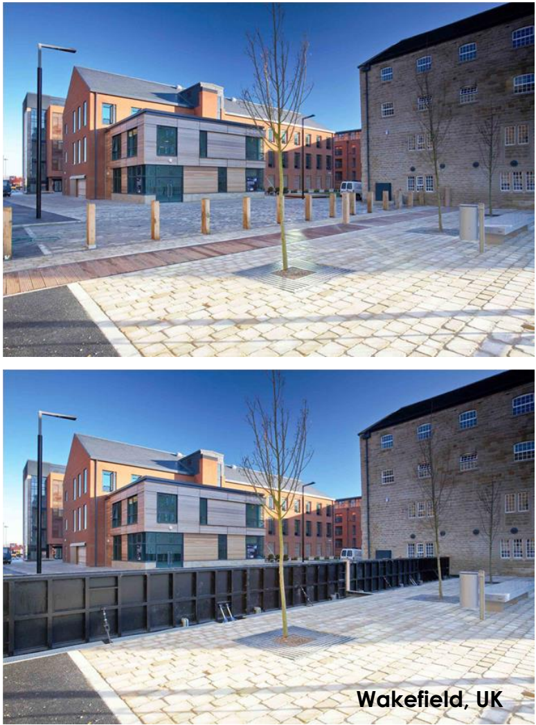
Flip-up flood barriers that can be remotely deployed and incorporated into the street (Image credit: Flood Control International)
