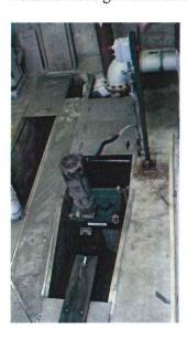
Influent Pumps – The influent pumps are included in the headworks building. Due to the high variability of the flow (low in summer and high in spring), the influent pumps operate a large portion of the year at low flow or high flow. It would be helpful to the overall operation of the plant if the influent pumps could be redesigned to provide the ability to function properly with low and high flows.
