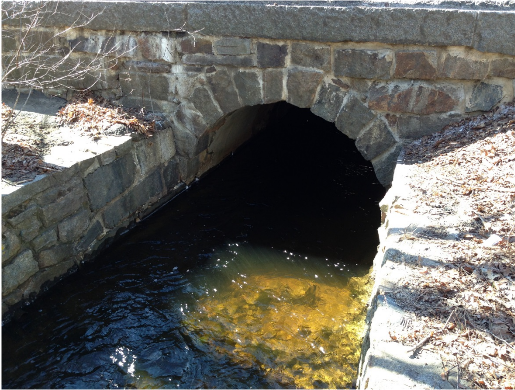
Photo 7: The upstream side of the School Street culvert is an example of the narrow, channelized character of Sawmill Brook. This location overtopped in the 2006 Mother's Day storm, causing extensive damage to adjacent properties. The gravel bottom and location just upstream from Central Pond provides a prime rainbow smelt spawning location.
