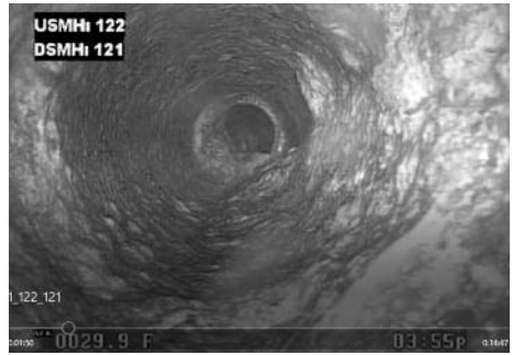
Cast Iron Sewer Pipe Before CIPP Lining
