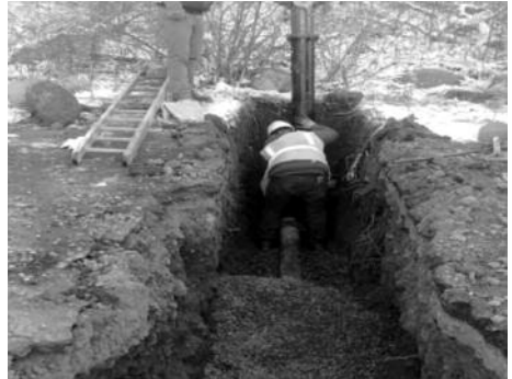
New Fire Hydrant Being Installed
